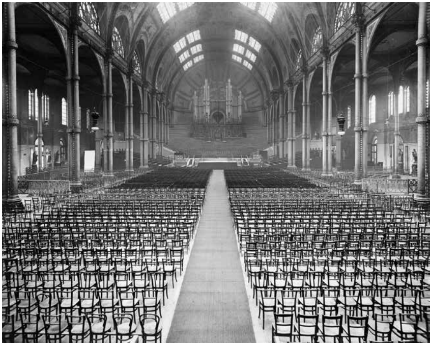
A long shot of the hall from the clock at the rear. This shows the roof and the side aisles off superbly. There appears to be various statues down the sides of the aisles, making the hall feel somewhat ecclesiastical.
